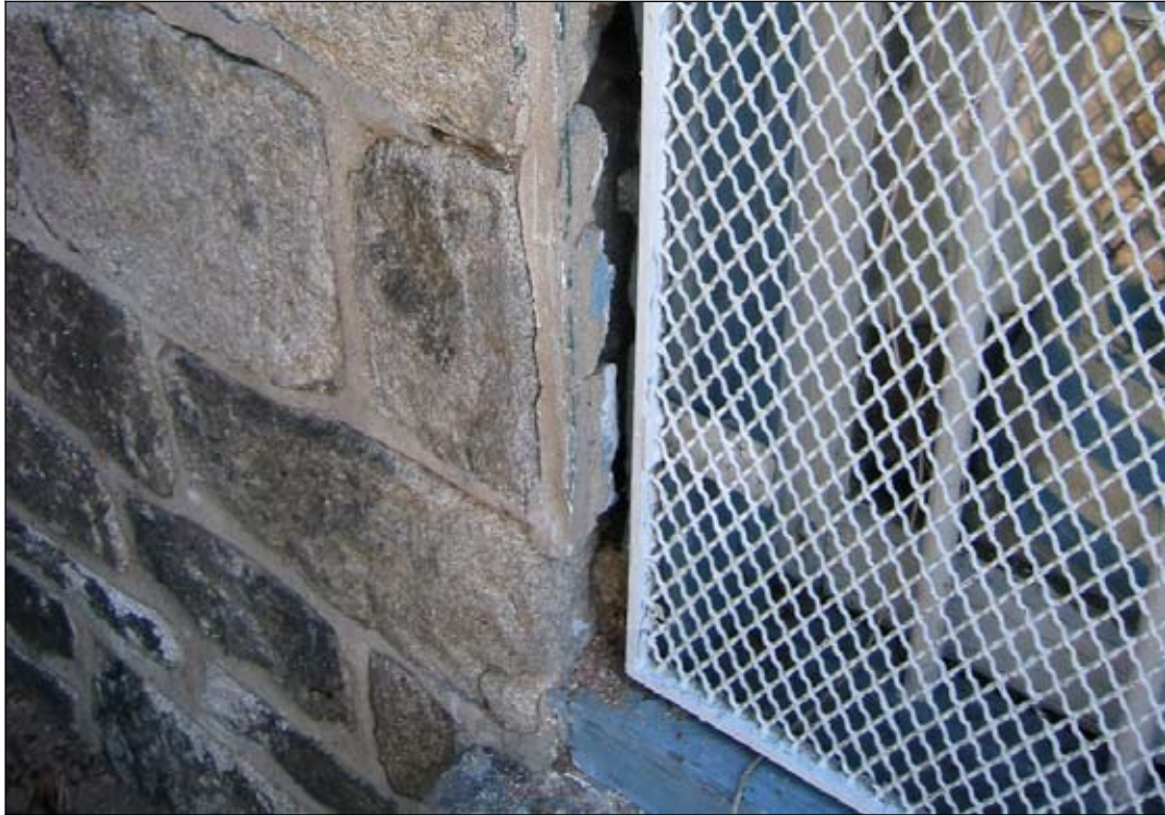
Figure 27: West elevation, detail of basement window where the mortar sample was taken. (Photograph by author, 2005)
