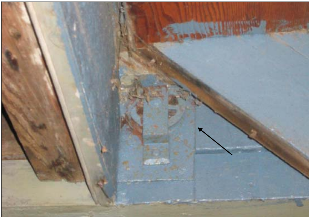
Figure 16: Metal pulley at top of basement stair, shows evidence of rope and pulley system. (Photograph by author, 2005)
