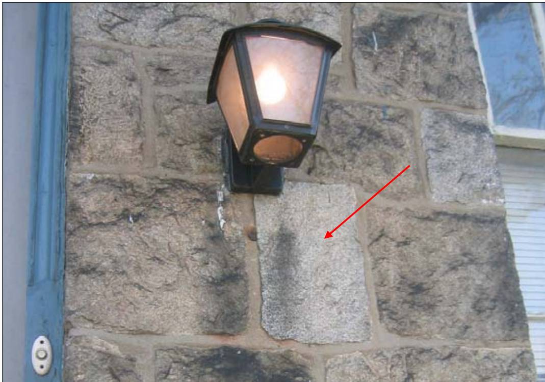
Figure 49: North elevation, detail. View shows staining of stone underneath the iron lamp, most likely due to the metal's chemical reaction with water from rainfall.
