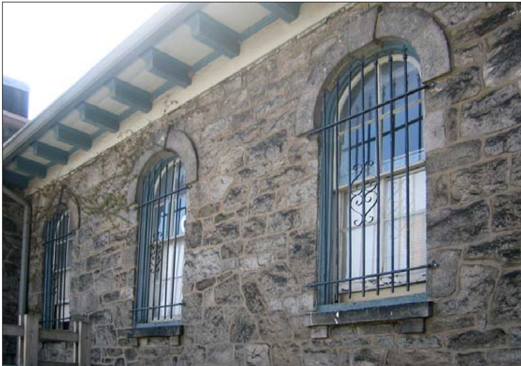
Figure 57: East elevation, detail. View shows iron rod grilles over window openings.
